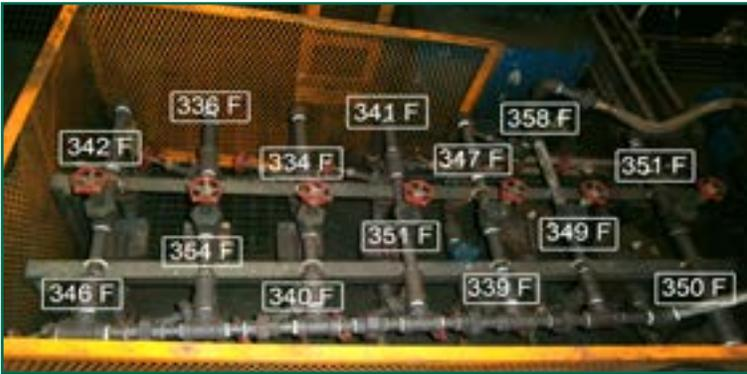
*Photographs can be used to document certain machine conditions. A picture of a set of steam traps with inlet and outlet temperatures can show they are working properly.*
