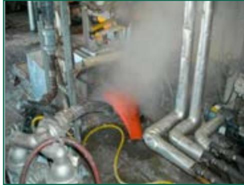
**A** bad Johnson joint on a single facer can be shown spewing steam out of the vessel, thus allowing maintenance to prepare adequately to fix the leak. Pictures of bearings expelling metal shavings versus a blown race, will help maintenance determine the urgency of a repair and avoid unwanted downtime.
