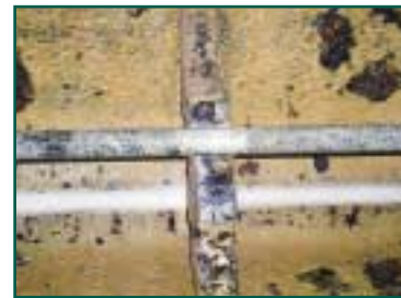
Center bearing missing
