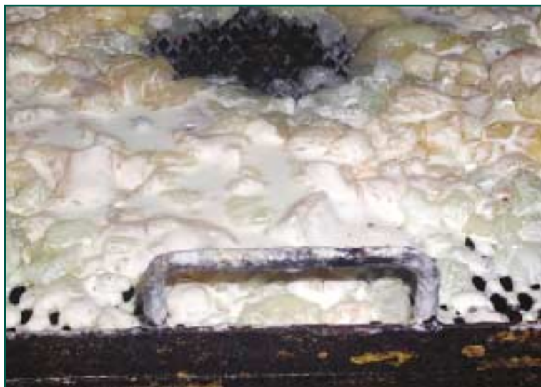
Starch strainer full of debris
