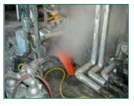
A bad Johnson joint on a single facer Acan be shown spewing steam out of the vessel, thus allowing maintenance to prepare adequately to fix the leak. Pictures of bearings expelling metal shavings versus a blown race, will help maintenance determine the urgency of a repair and avoid unwanted downtime.
